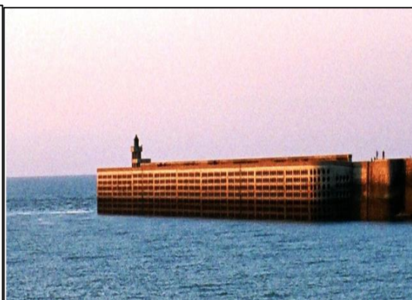
Perforated front wall breakwater
