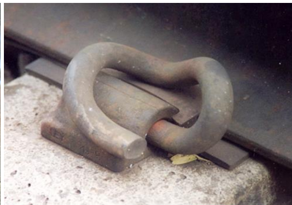
Pandrol clip fixed to rail seat
