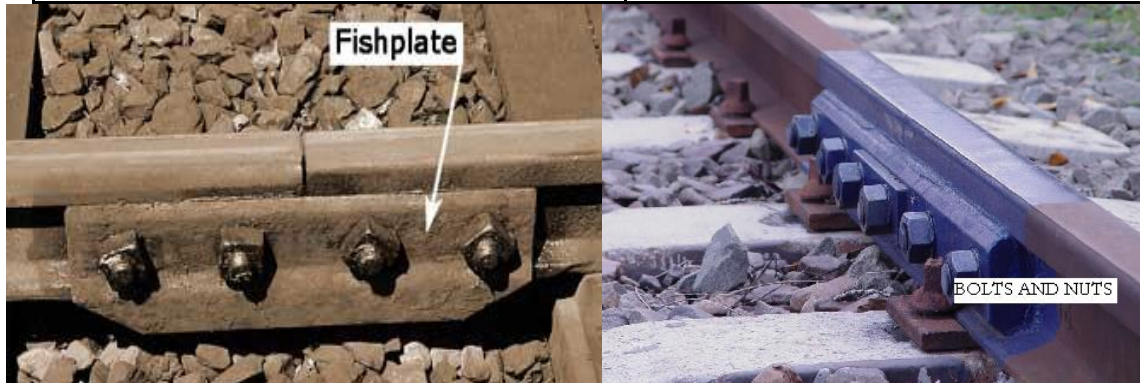
Fish Plates, Nuts and Bolts
