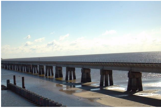
Piled breakwater with concrete wall
