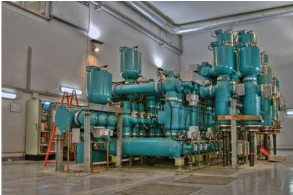
Gas Insulated Substation
